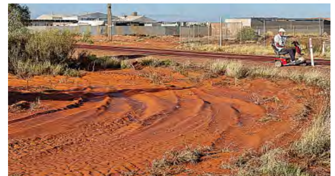
Sunday morning after continuous overnight rain, the culvert is completely concealed by mud.
