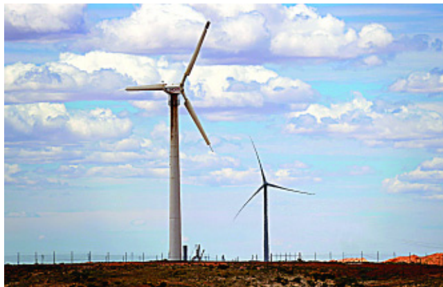
3) On the 19 January the blades appeared on SENVION wind turbine no 1 (REAR). The older NORDEX wind turbine in the foreground showing signs of wear and tear.
