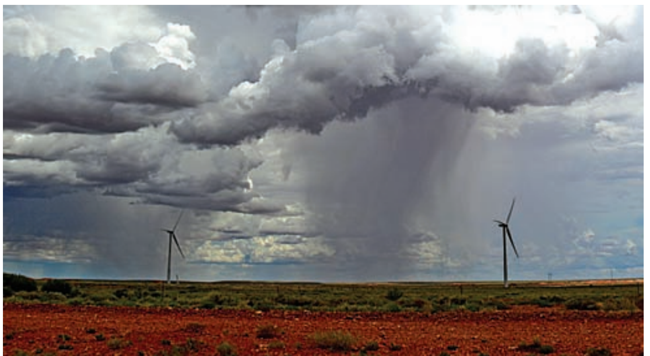
5) The two SENVION wind turbines were only just completed before a major rain storm hit the town.
