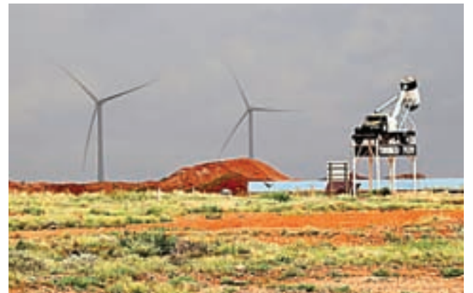
By the 23 January both SENVION wind turbines were upright with rotor blades intact
