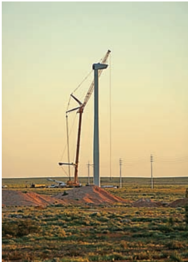
2.) By the 15 January the nacelle had been fitted to the mast of wind turbine no 1 with most of the working activity occurring at night due to weather conditions - mainly heat but sometimes rain or wind was a hinderance.
