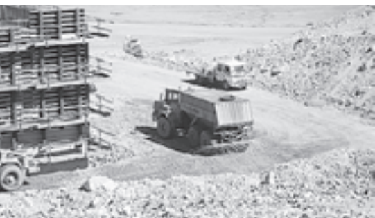
Left: Site construction in progress
